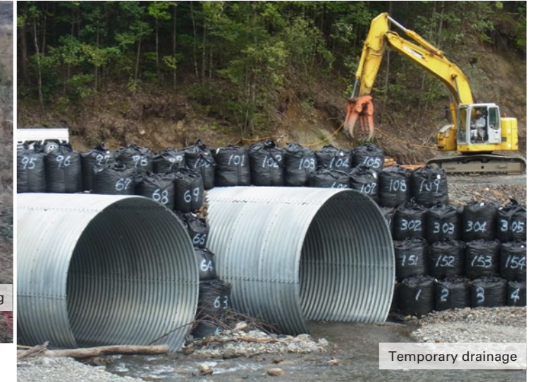
Temporary waterway tunneling
