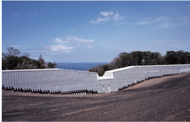
"SB WALL™ Construction Method"- An impermeable check dam constructed by using displaced soils at the construction site
