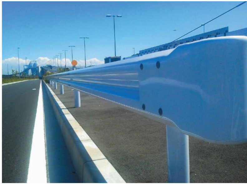
"Guardrails" are a typical product used as protective fences for vehicles, and are widely used from high-standard highways to general roads. The wave-shaped beam cross section offers excellent line-of-sight guidance.
