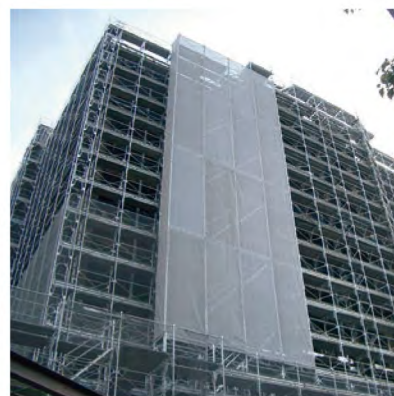
Frame type Scaffold
