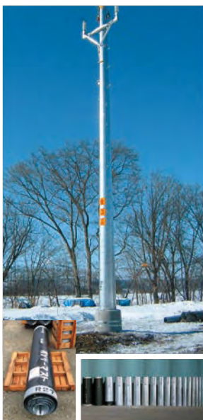
Transmission / Distribution line mast
