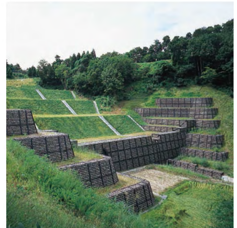
Steel Frame Dam
