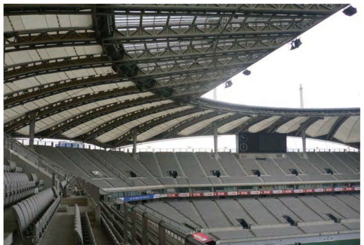
Truss structure roof using LGS
