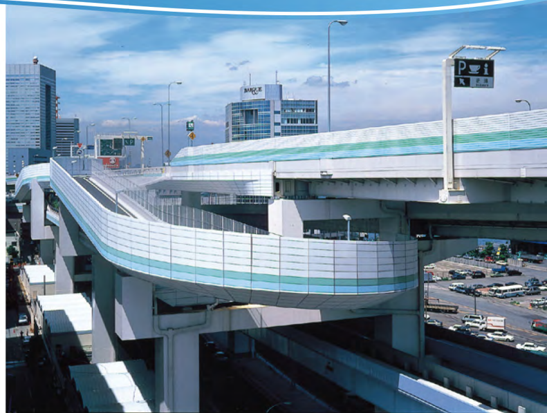
Noise Barrier for highway
